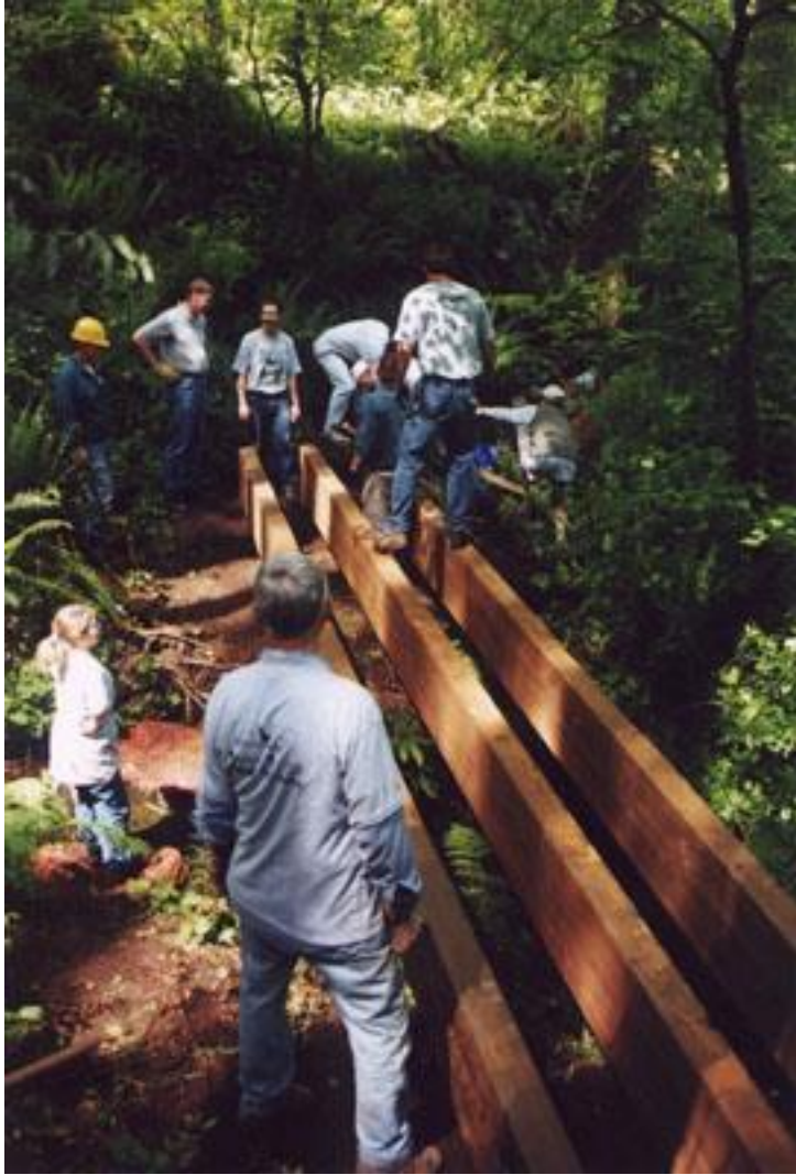
The crew is setting the large pressure-treated stringers that will support the bridge decking.
