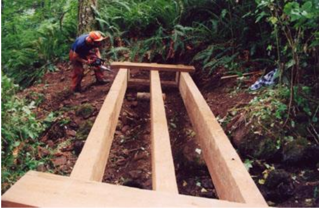
A gasoline powered drill is being used to bore holes in the stringers for the bridge.
