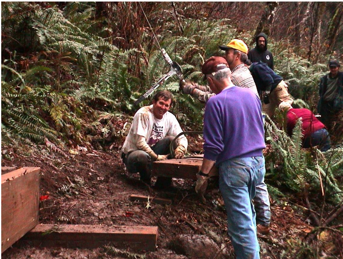
This is preliminary work on the third stringer.
