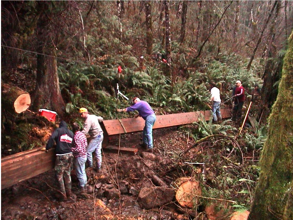
The crew is using a highline to “fly” the stringers in place. Jerry deRuyter set the highline for the bridge work.
