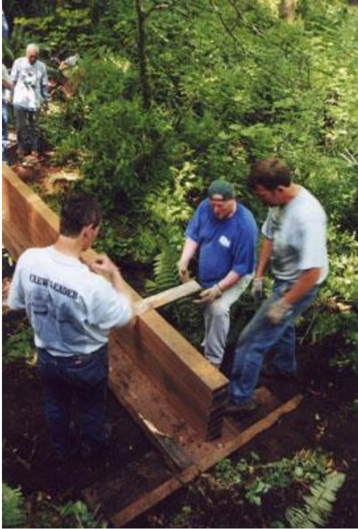
The crew is checking the first stringer for placement.
