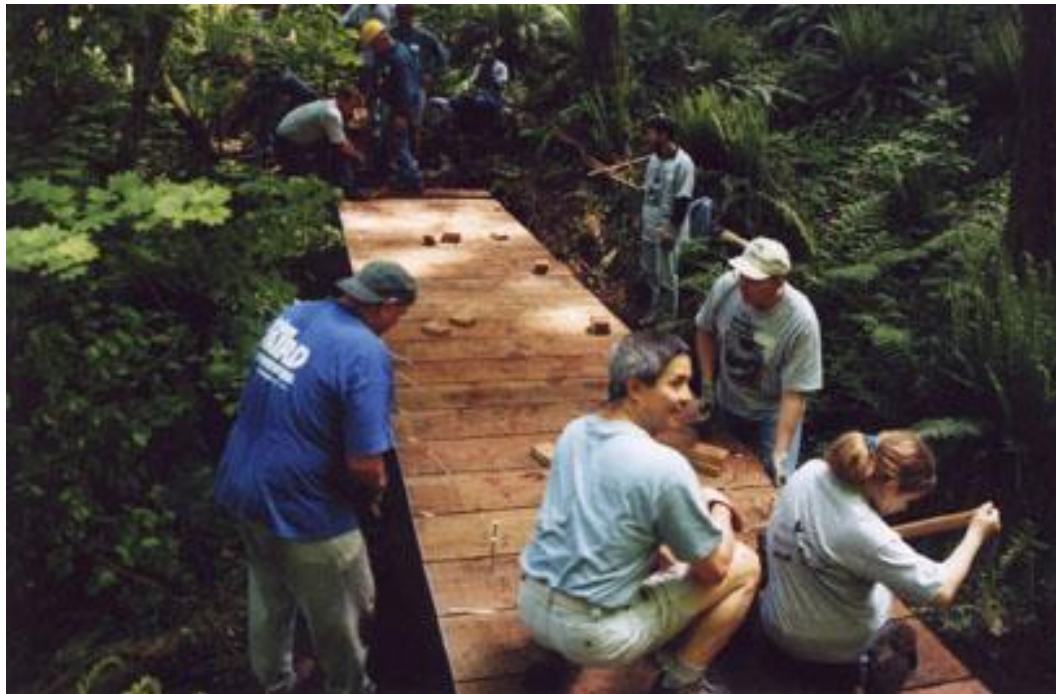
Craig Pridemore is helping to construct the bridge. The bridge decking is done and the crew is preparing to install the kick rail.
