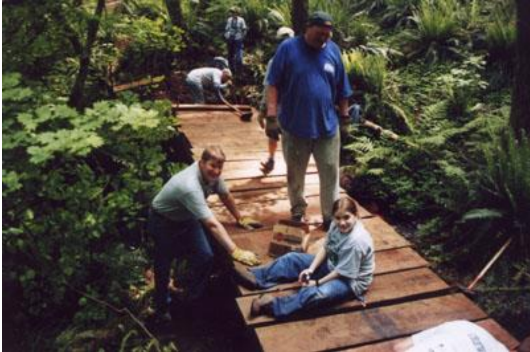
Putting the decking on the bridge. you can see the decking is still loose.
