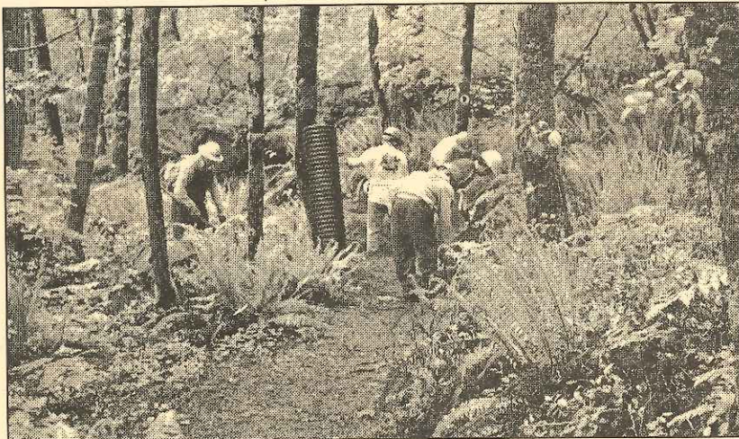
NTD trail workers installing culvert
