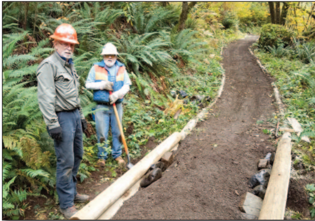
Replacing the Trail Timbers
